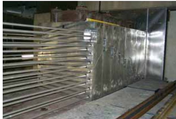
NuMI downstream absorber. Note elaborate cooling. “Cost more than NuTeV beamline...” – R. Bernstein
