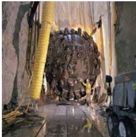
NuMI tunnel boring machine. 3.5yr civil construction
